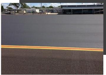
FRM SealCoat is a plural component, single package, reactive, high molecular weight polymer modified bitumen sealcoat. FRM SealCoat is designed to penetrate deep into pavement substrates where it permanently weather seals airport, street and highway apron surfaces. It may be applied as a mineral filled sealer through spray, broom, or squeegee and may be applied as an un-filled coating through high volume equipment.
