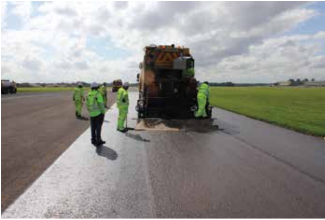
Application of 5mm Microsurfacing on existing Asphalt
