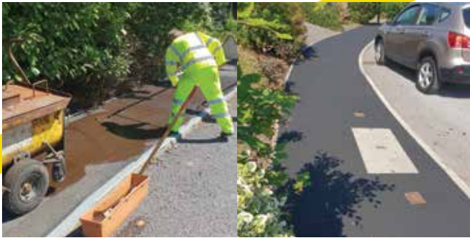
Before & after hand applied footway Microsurfacing
