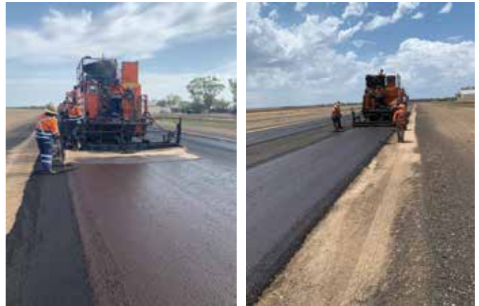
During application of Colmat 7mm
